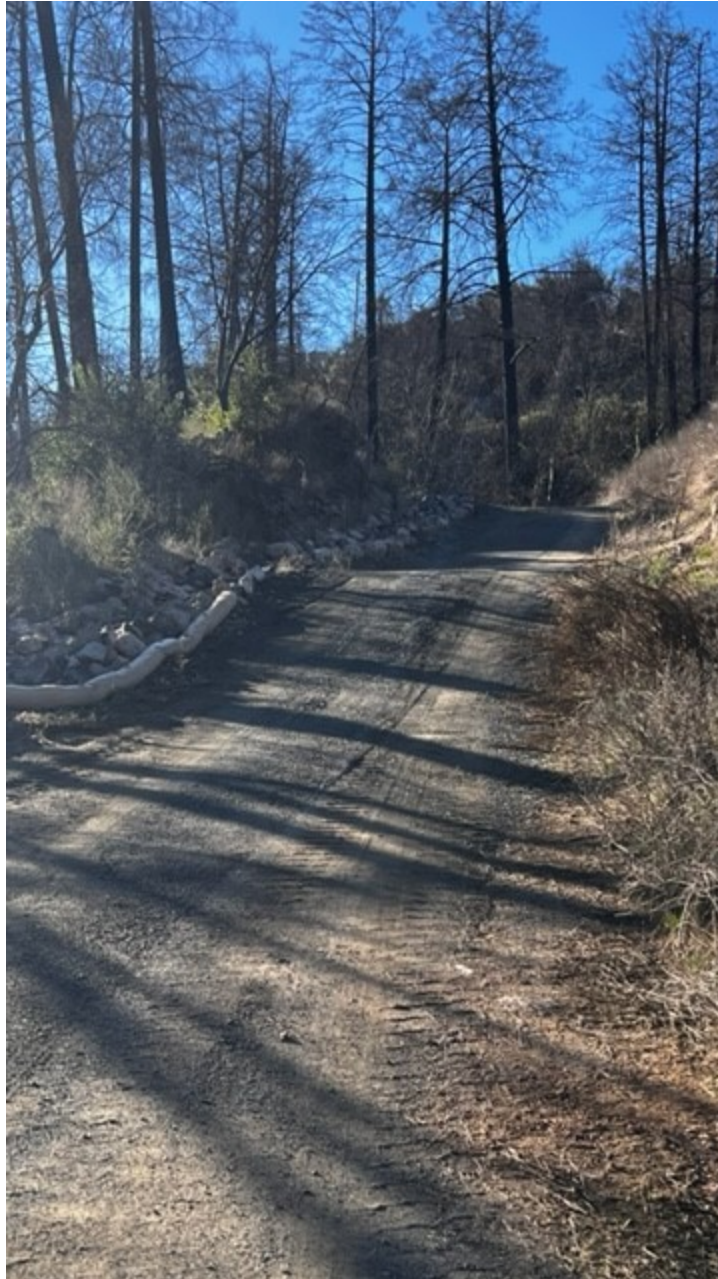
Water bars, rip rapped drainage channel, and fiber rolls on southern access road to SL-4
