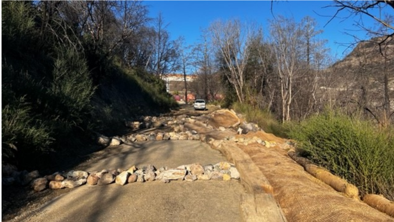
Rock water bars, geotextile matting, fiber rolls, and gravel along SL-5A access road.
