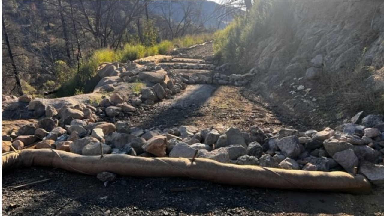
Water bars along SL-5A access road
