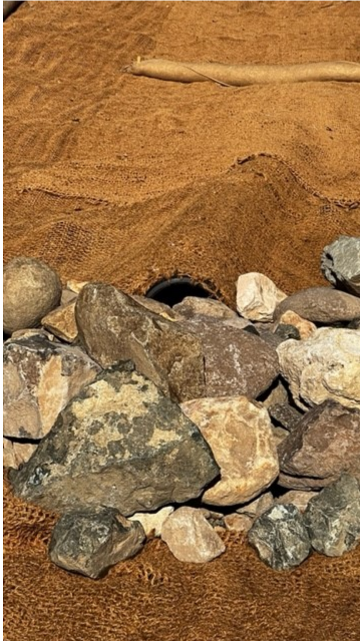
Mouth of drain pipe and riprap on northern access road to SL-4
