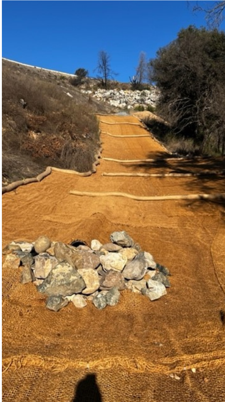
Fiber rolls, jute netting, filtration netting, drain pipe, and rip rap on northern access road to SL-4
