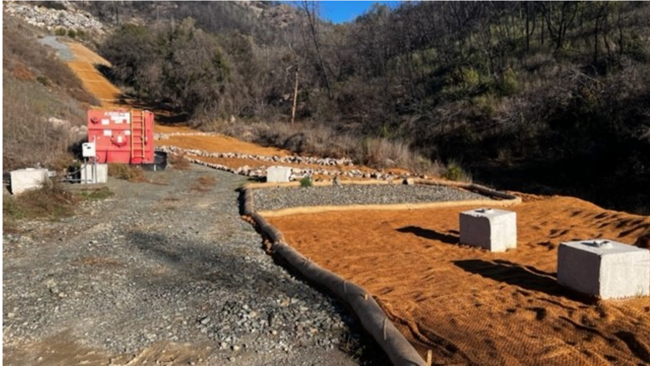
Fiber rolls, jute netting, filtration netting, rip rap, rock water bars, and gravel at SL-4
