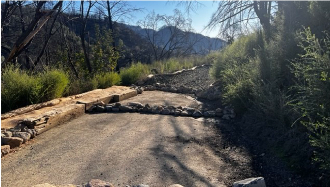
Rock water bars, fiber rolls, and gravel along SL-5A access road.
