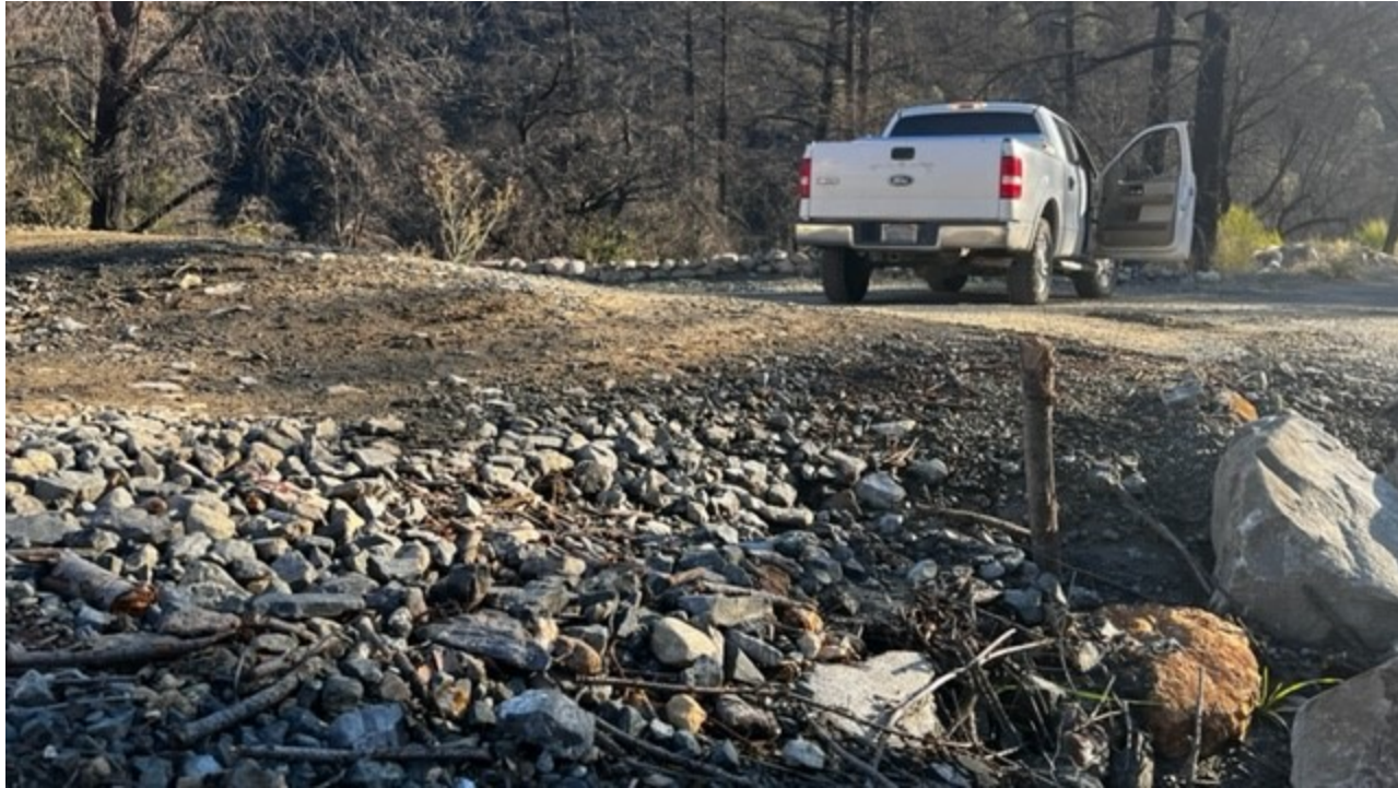
Water bar on southern access road leading down to SL-4
