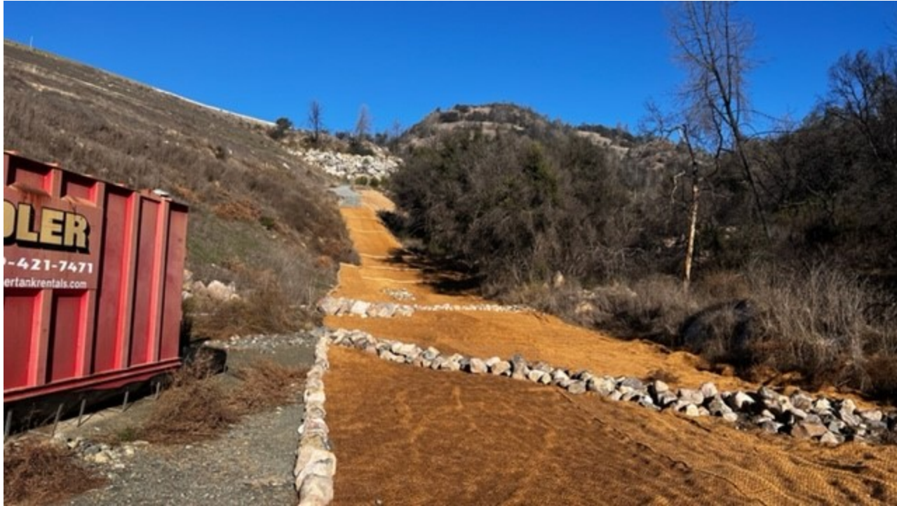
Fiber rolls, jute netting, filtration netting, and water bars on northern access road to SL-4
