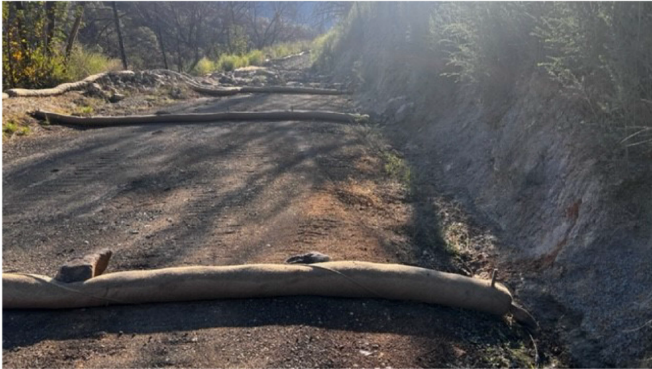
Fiber rolls along SL-5A access road
