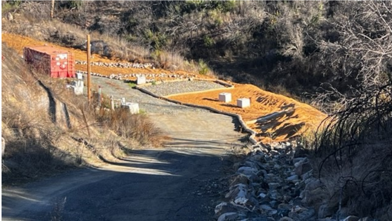
Fiber rolls, jute netting, filtration netting, rip rap, rock water bars, and gravel on southern access road to SL-4
