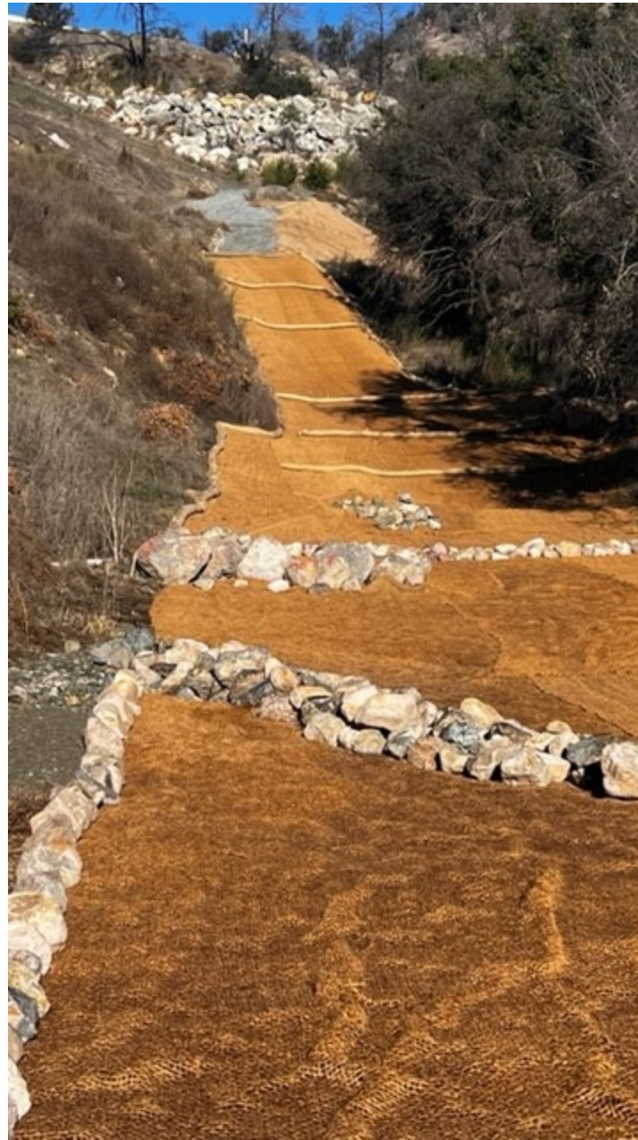
Fiber rolls, jute netting, filtration netting, and water bars on northern access road to SL-4
