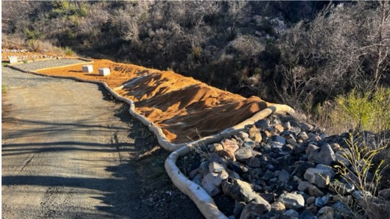
Fiber rolls, jute netting, filtration netting, rip rap and gravel on southern access road to SL-4
