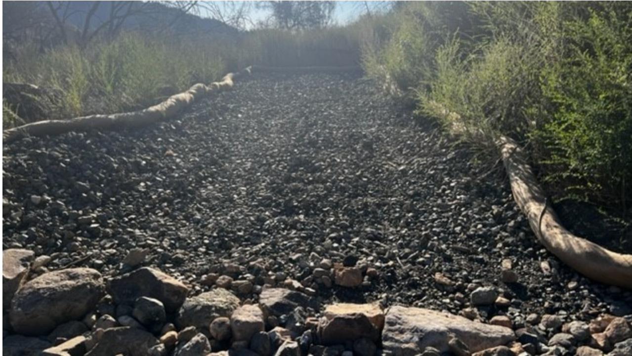
Settling bed used to settle out sedimentation on SL-5A access road.
