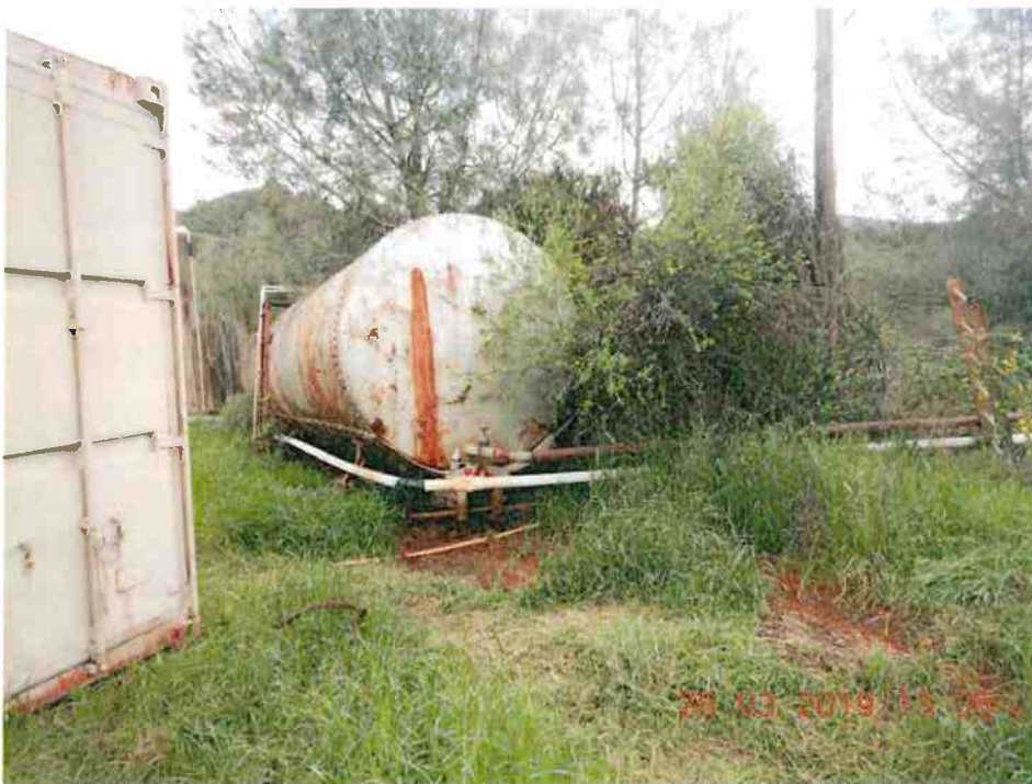
Photo 521- rust staining and leakage from the leachate condensate tank, looking northeast.
