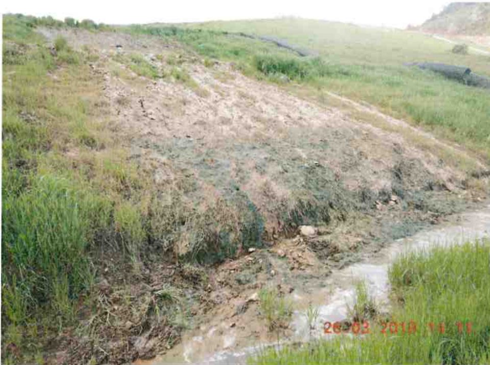
Photo 615- erosion from stormwater and leachate overflow, leachate ponding on the bench, looking northwest.
