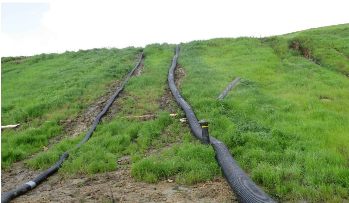
Figure 4. Looking upslope toward active landfill (not in view). Black plastic storm drain pipe on right originating from landfill travels down slope into Stream 1 (March 28, 2019) (Allen 2019).
