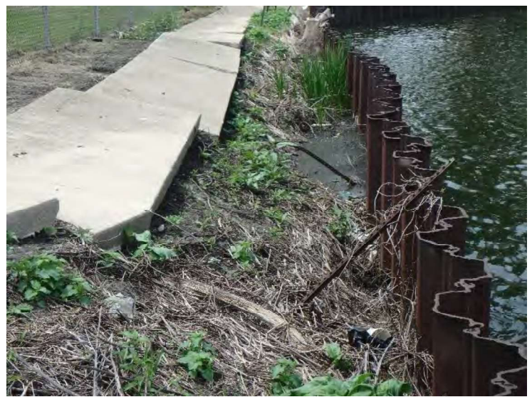
Washed out backfill at Sta. 12+00
