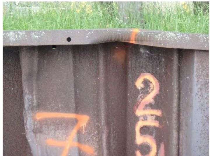
Area of impact damage at Sta. 7+00
