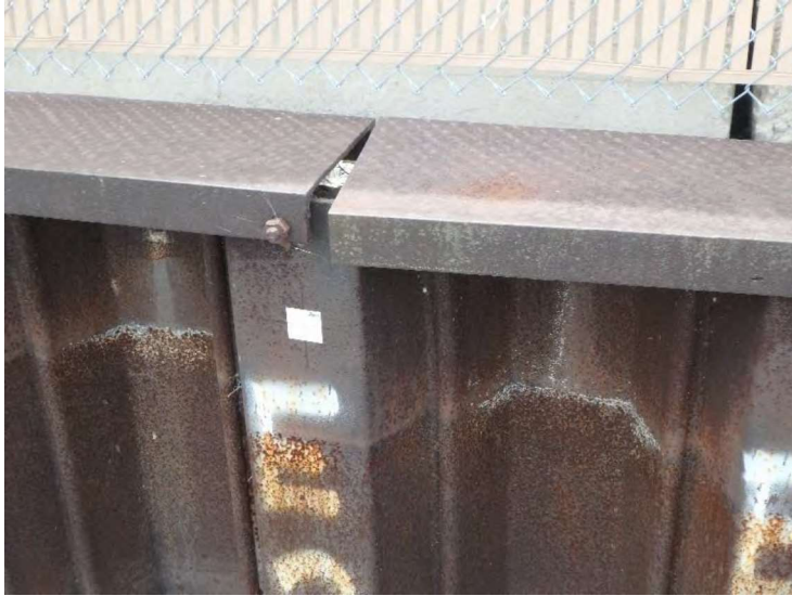
Bulkhead leaning outward and separation in the cap at Sta. 3+95
