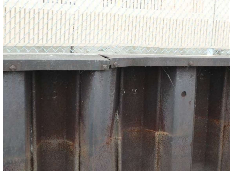
Area of impact damage at Sta. 4+90
