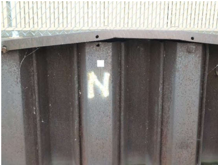
Cap deflected upward at Sta. 6+00
