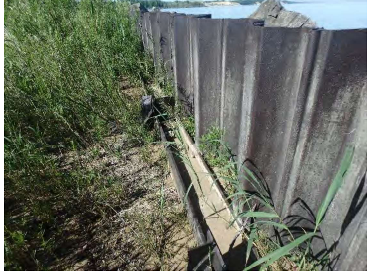
Typical condition of tiebacks and wales on the outer bulkhead
