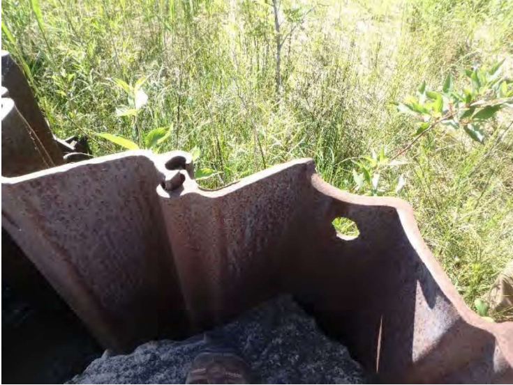
Typical impact damage due to driving on the outer bulkhead
