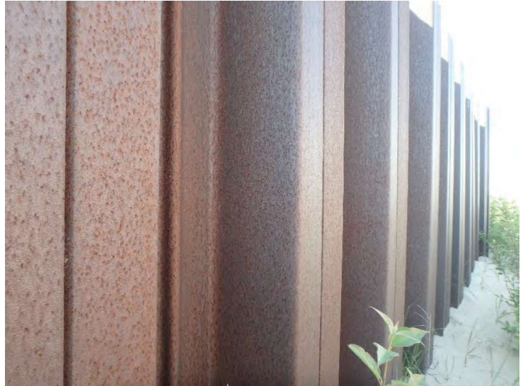
Typical inner bulkhead sheet pile condition
