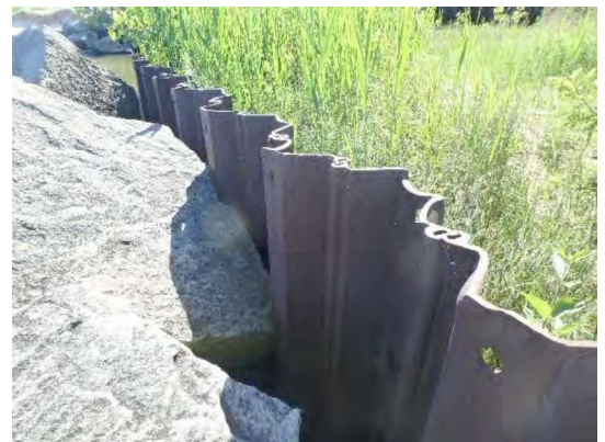
Typical outer bulkhead sheet pile condition above water
