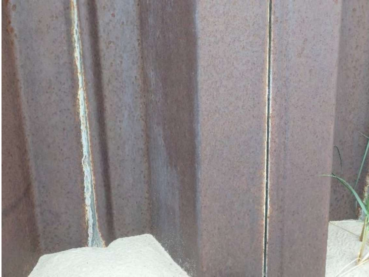
Typical seepage through the sheet piles on the inner bulkhead
