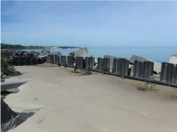
Removed sheet piles on the outer bulkhead for drainage
